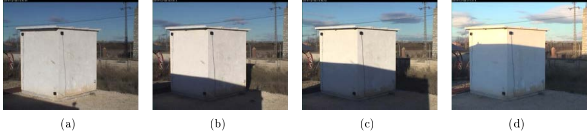
Figure 3.14: The presence of other buildings shadowing the sunshine introduces largely different on-board temperature profiles among different wireless sensor nodes.
